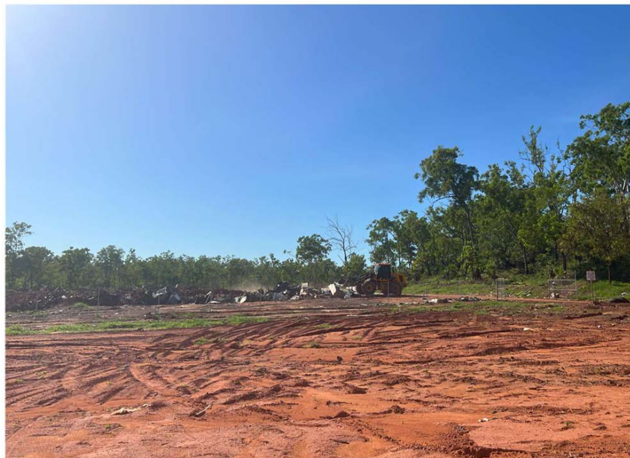
Figure 4.4 Landfill Operation in Wadeye Waste Management Facility
