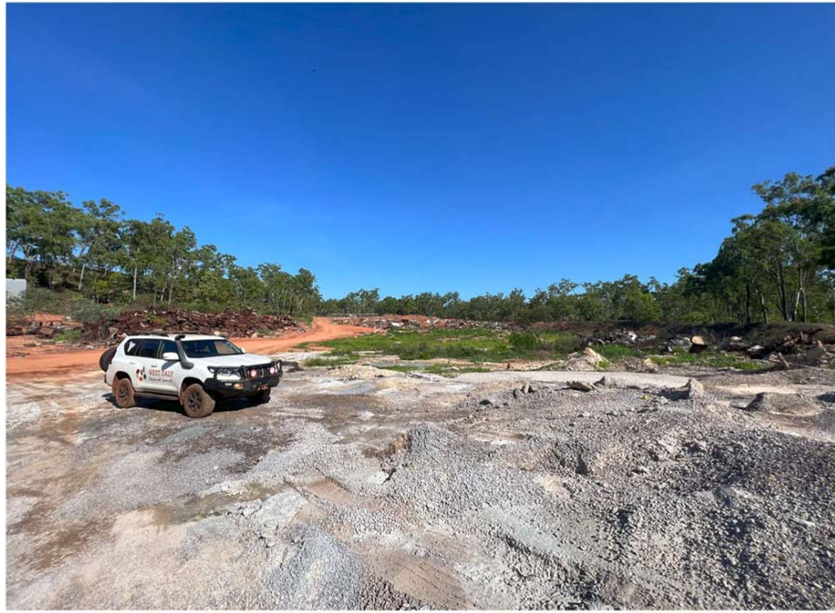
Figure 4.3 Concrete Wash Down Area in Wadeye Waste Management Facility
