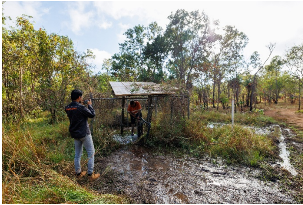
Koy – Water Bore repairs
