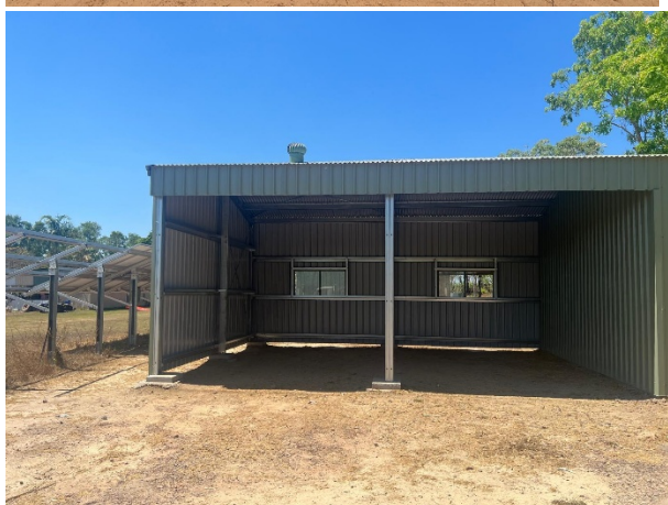
Merrepen New Shed & Uminyuluk New Shed
