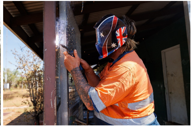
House repairs – Old Mission
