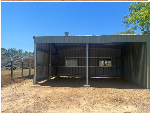
Merrepen New Shed & Uminyuluk New Shed
