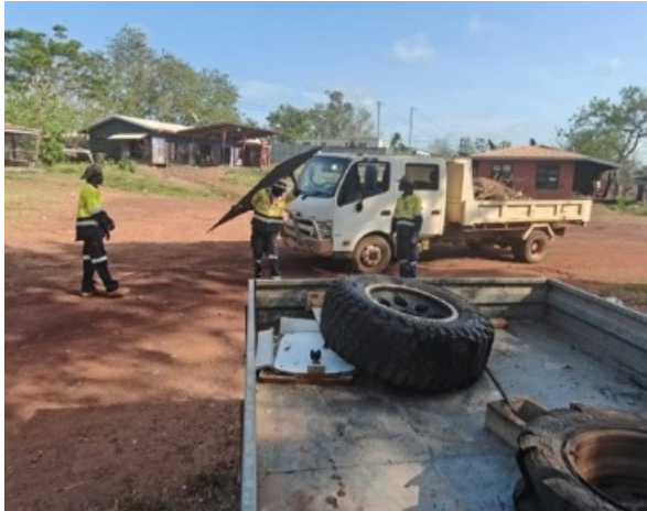
Wadeye civil works team -clean up works bottom camp
