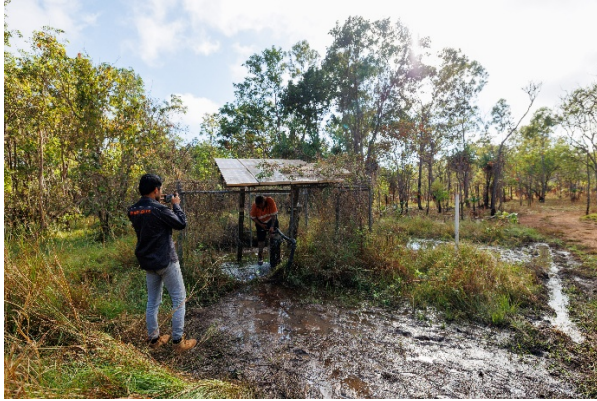
Koy – Water Bore repairs
