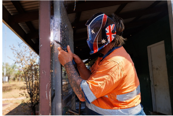
House repairs – Old Mission
