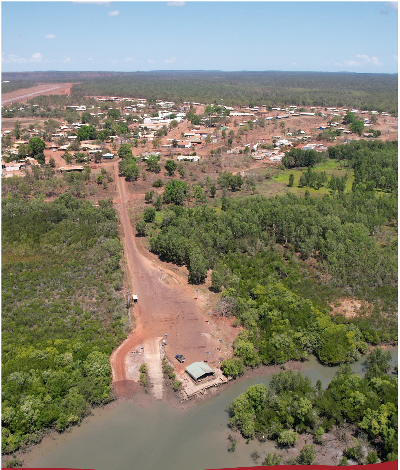
Wadeye barge landing
