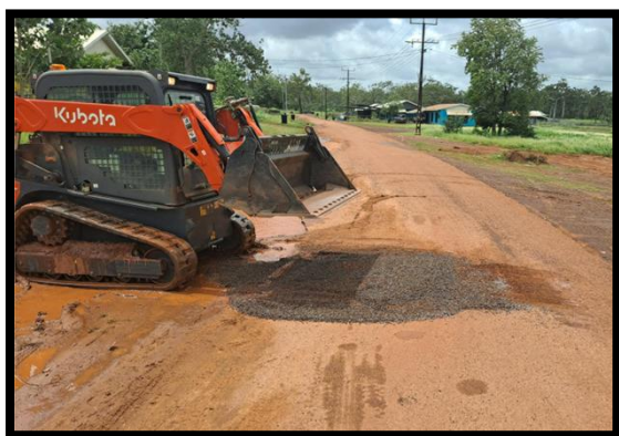
Kolumboort Street - Pothole patching
