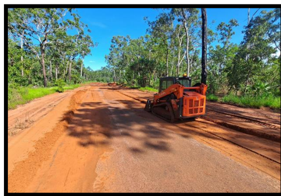
Wadeye-Manthathpe Road – Road maintenance works
