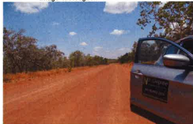
Image 2: Hodgson River Rd - Site Visit
