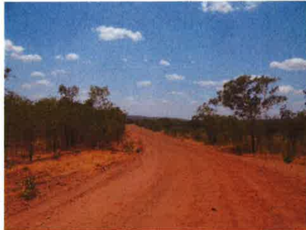
Image 1: Hodgson River Rd - Site Visit
