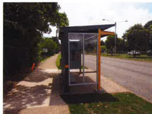
Image 2: Landed bus shelter Trower Rd
